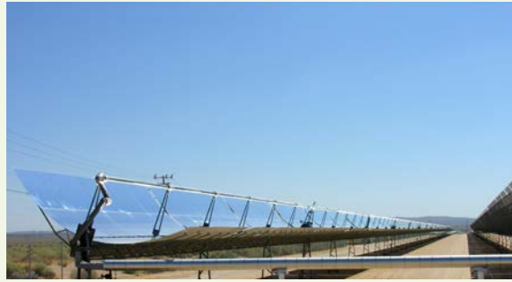
Figure 25.44 Parabolic trough collectors are used to generate electricity in southern California. (credit: kjpg, Wikimedia Commons)
